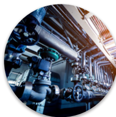
Oil Tank Rooms
